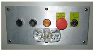
Key switch: Turn on to activate landing buttons (1 or 2) Landing buttons (I or II): Press to move platform to desired landing 1 or 2 Emergency stop: Press to stop the platform immediately (overrides the call stations and sounds the alarm) Alarm button: Press to activate alarm
